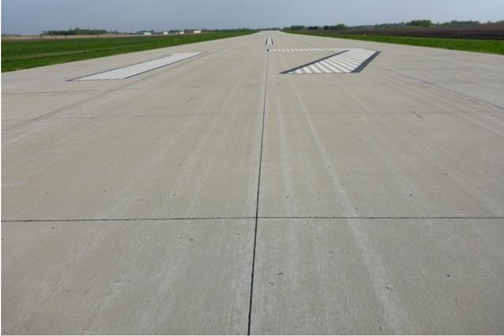
MWM RY1735 001 (PCI = 97)
