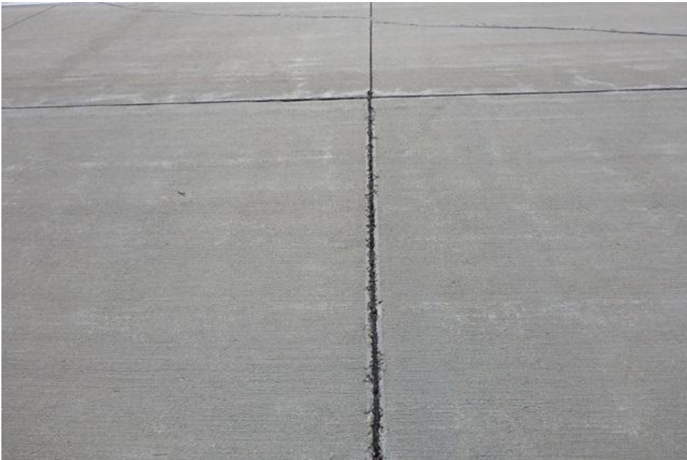
MWM RY1735 001 (PCI = 97)
