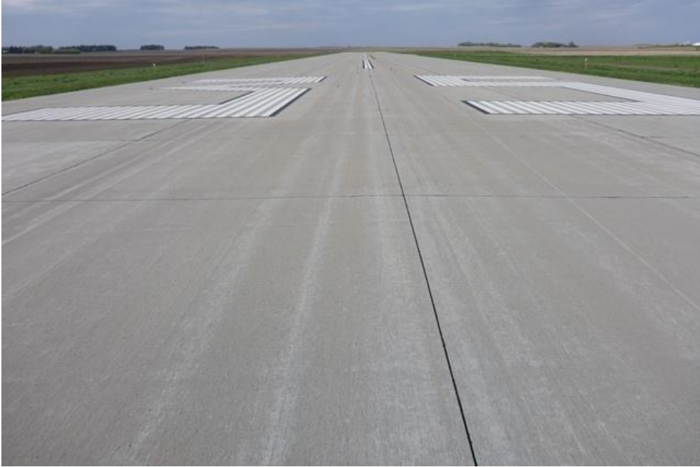
MWM RY1735 001 (PCI = 97)
